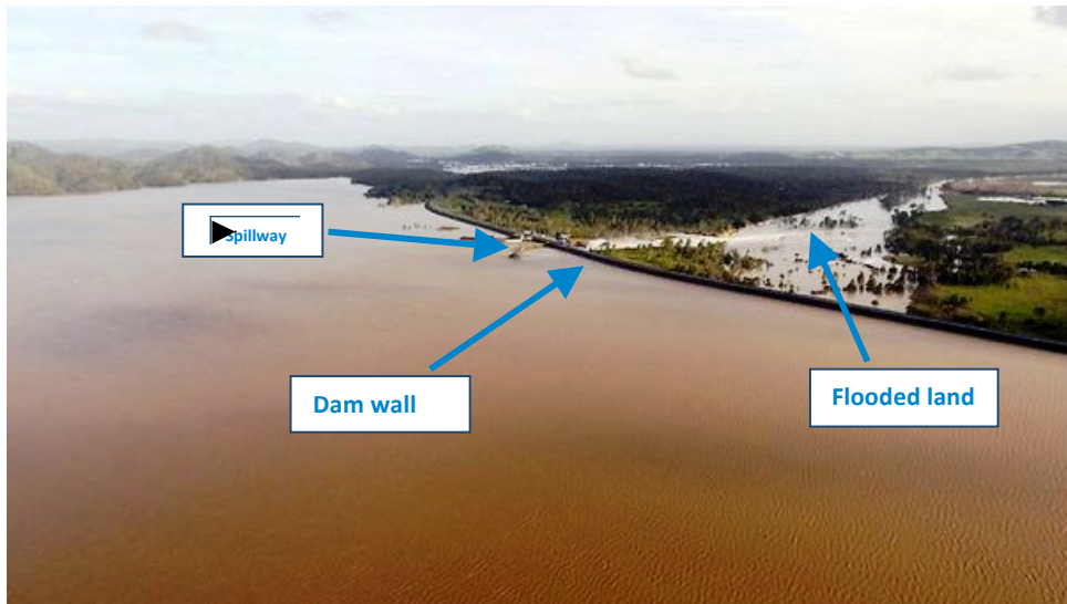
Fig 1. Wivenhoe dam, the main water supply for Brisbane, capital of Queensland during the peak period.
