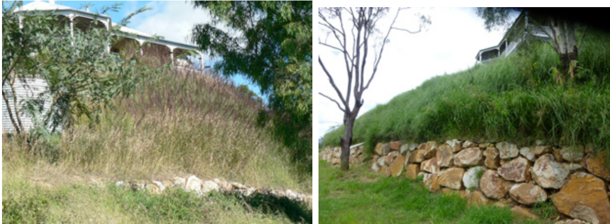
Fig. 14: The house was fully protected during the high and intense rain fall periods
