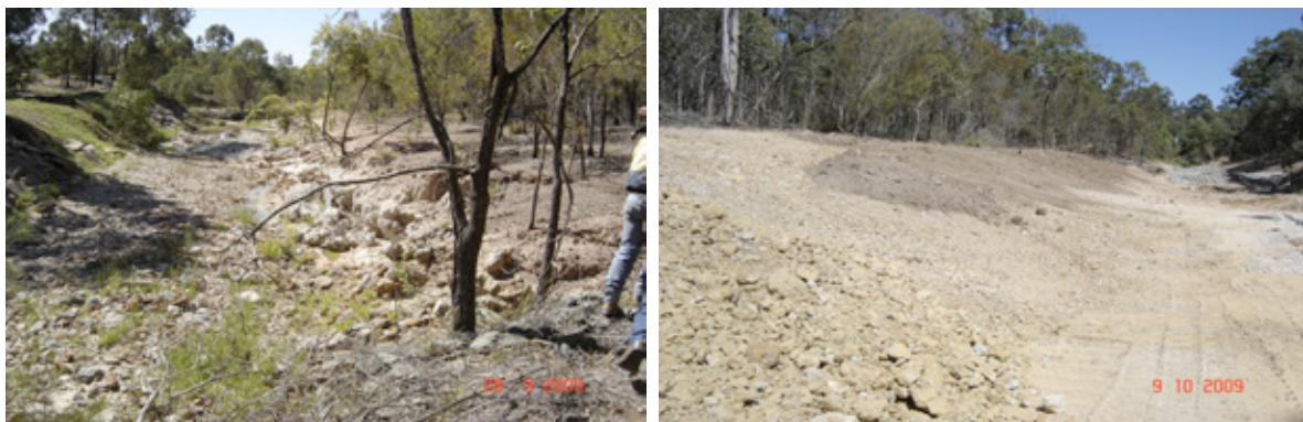
Fig 4. The drain before and after earth work prepared for vetiver planting
