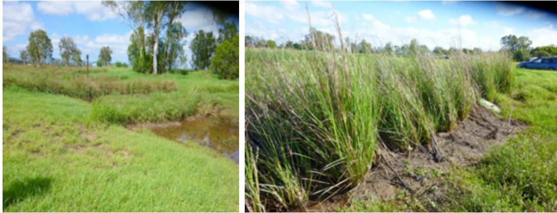
Fig 3. Very little damages to the vetiver rows and the catchment
