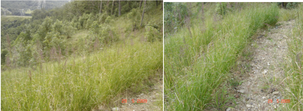
Fig. 16: The slope was fully protected during the high and intense rain fall periods in the next two years
