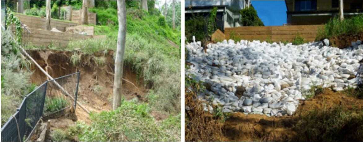
Fig. 8: Eroded riverbank threatened the foundation of the house and soil bags were used to fill the hole
