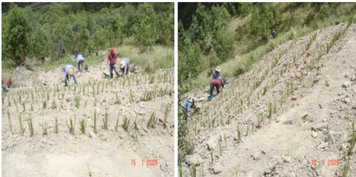
Fig. 15: Planting Vetiver following site reparstion
