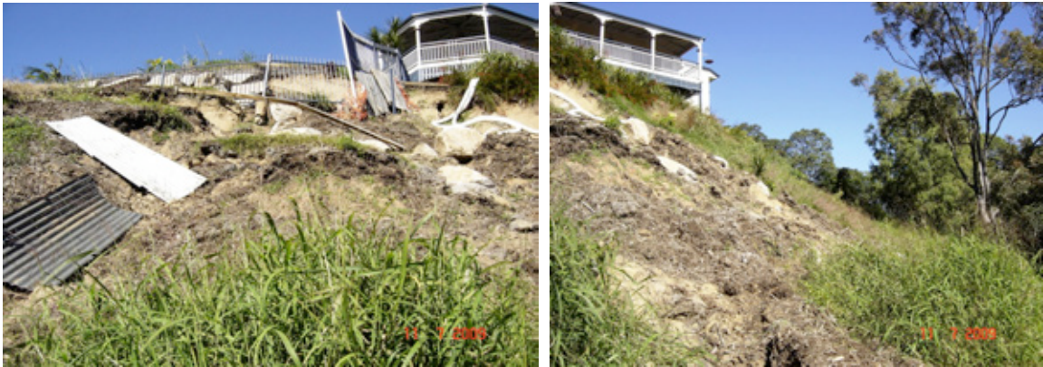
Fig. 11: Landslide threatened the foundation of this house on a very steep hill
