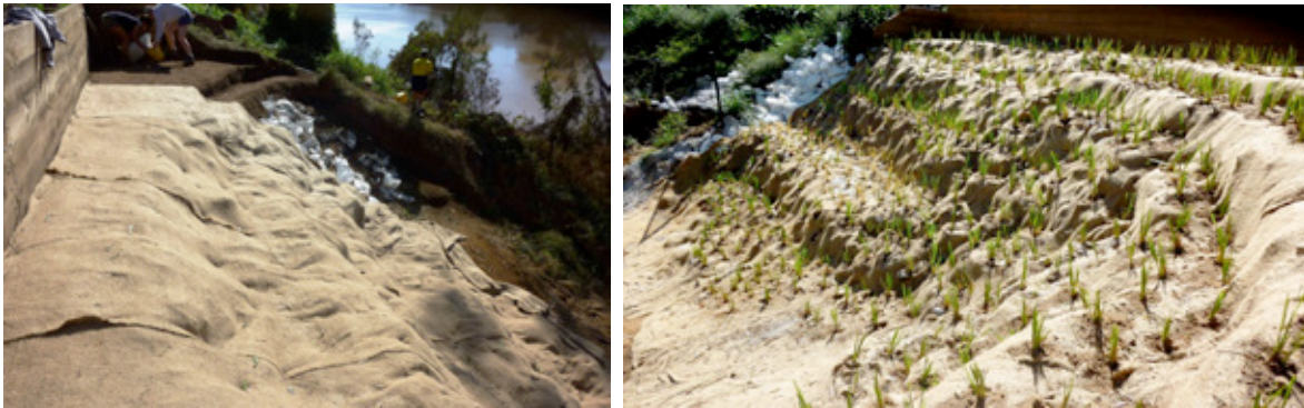
Fig. 9: Jutemesh was used to give the bags temporary protection against rising water before vetiver was planted
