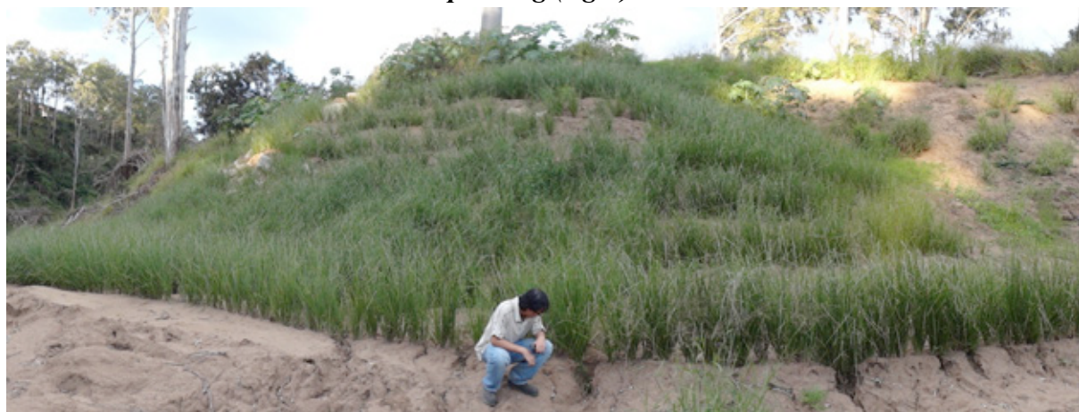
Fig 7. Three months after planting and has adequate protection against some minor floods
