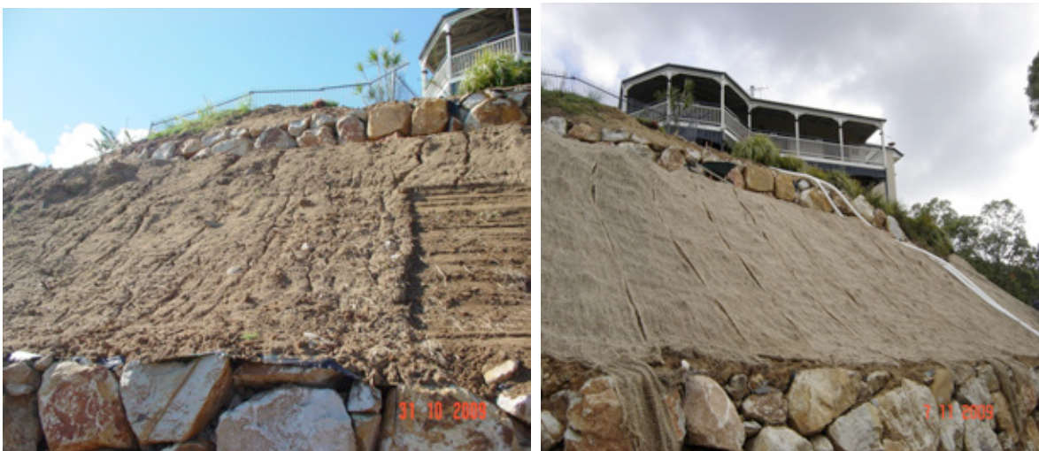
Fig. 12: The front slope after reparation and covered with jutemesh
